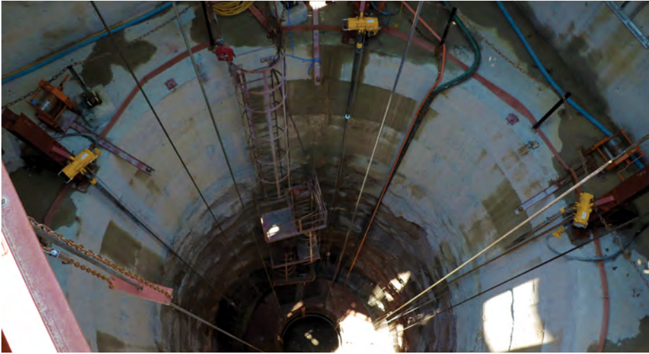
Start of Underground Shaft
